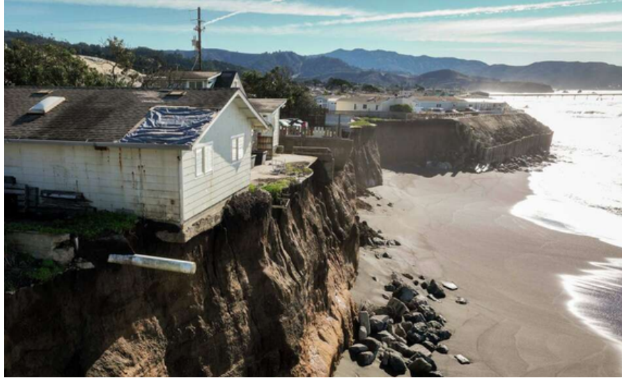
Home hangs over the edge of a cliffside impacted by erosion near Palmetto Ave in Pacifica, California (Bronte Wittpenn, SF Chronicle)
